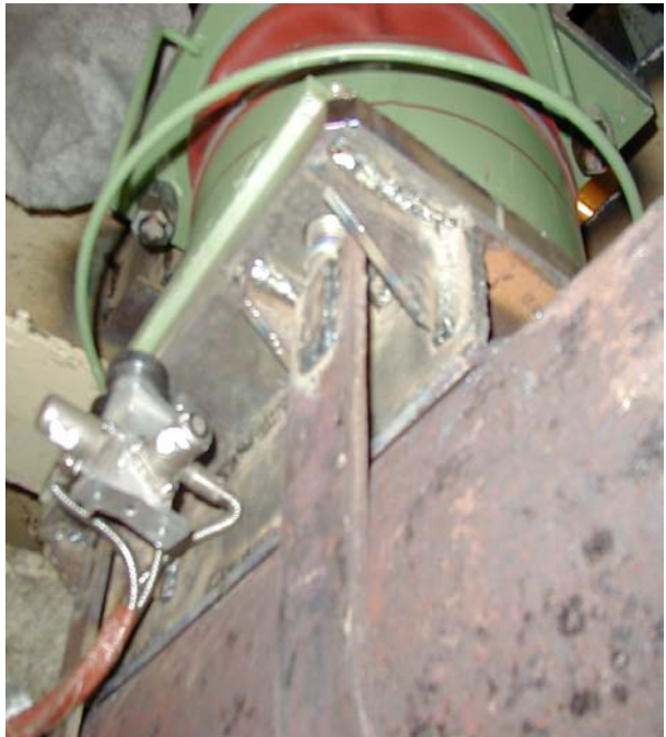
Figure 9. Installation of transducers on the damper's clamp on the piping 21.
