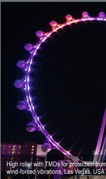
High roller with TMDs for protection from wind-forced vibrations, Las Vegas, USA
