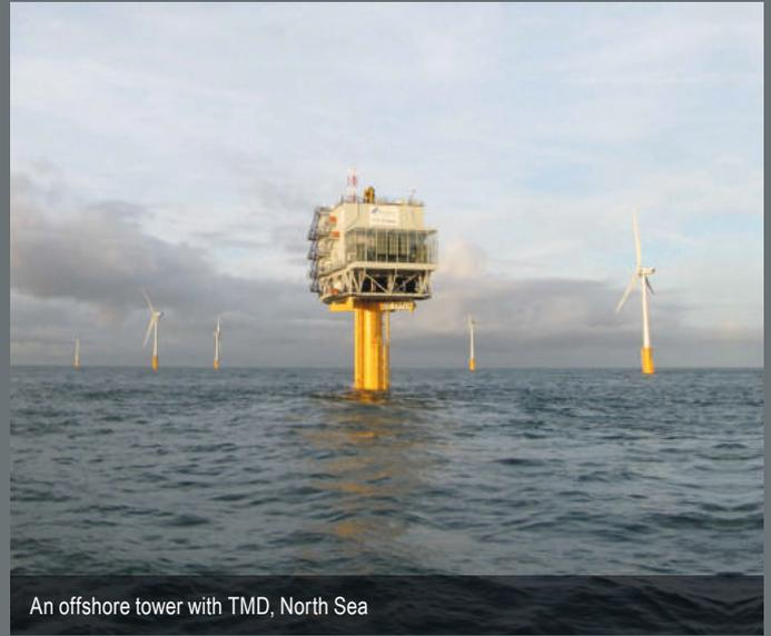
An offshore tower with TMD, North Sea
