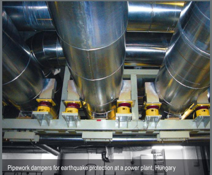
Pipework dampers for earthquake protection at a power plant, Hungary
