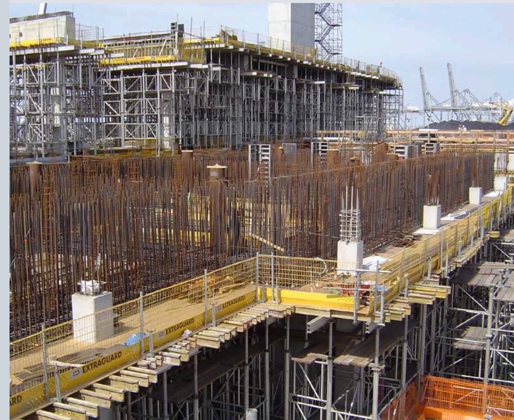
Construction of turbo/generator top mat – Rotterdam, Netherlands
