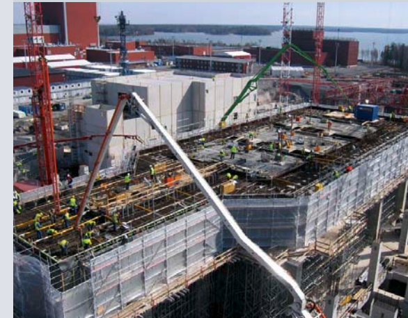
Pouring of concrete – Olkiluoto-3, Finland
