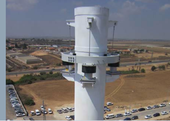
Stack with tuned mass damper
