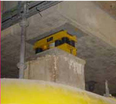
Retrofit of a Turbo Compressor Foundation, Germany
