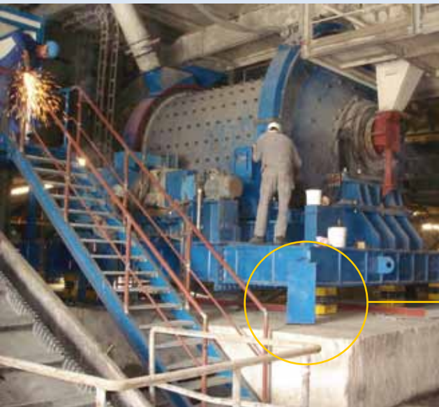
Retrofit of a Rod Mill, Germany
