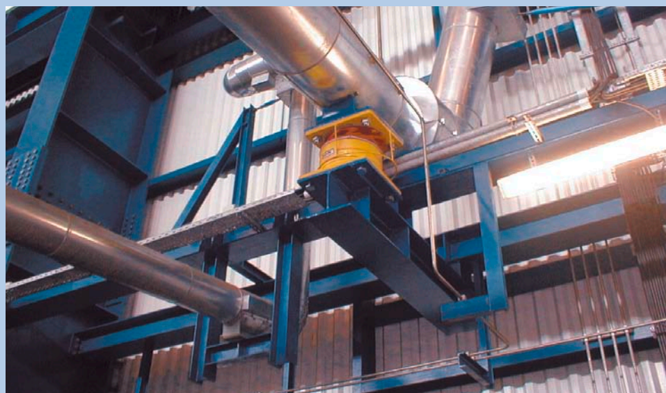
Installation of a pipework damper type VES
