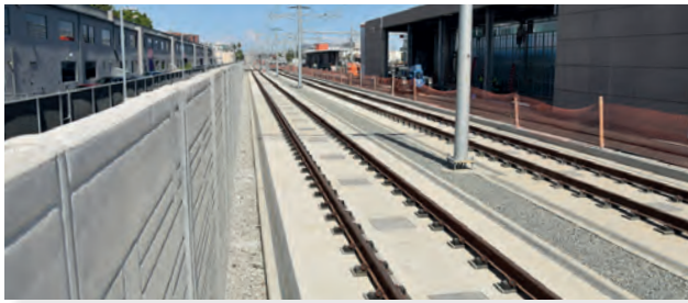
Steel spring MSS, Expo Line, Los Angeles, USA
