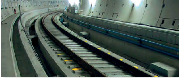
MSS with earthquake protection, subway, Tokyo, Japan
