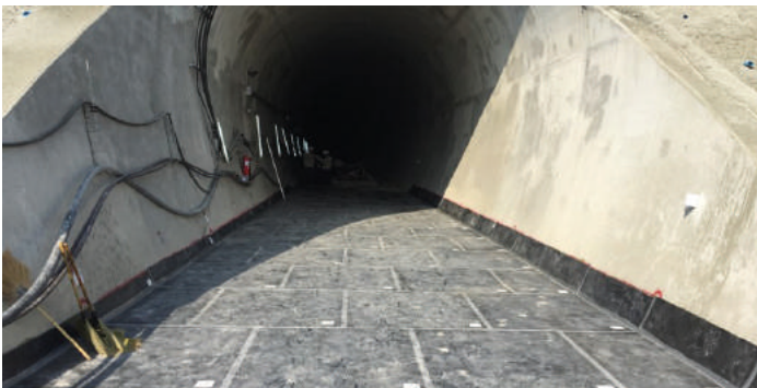
Tunel Phra Puttachai | NOVODAMP® MAT, Tailandia
